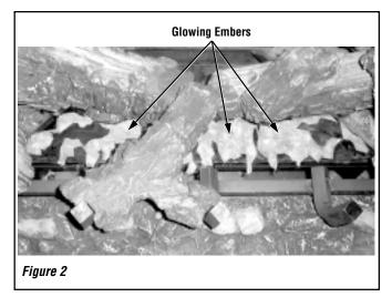
Proper log placement is critical to encourage outstanding flame appearance and prevent sooting. When positioned properly as shown, logs will be positioned between flame peaks and will not impinge any flames.
